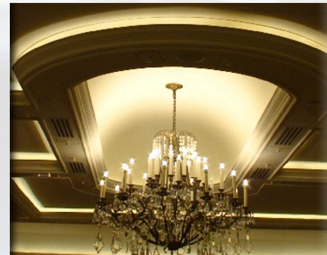
Custom GRG Race Track Dome San Antonio Country Club Ballroom
